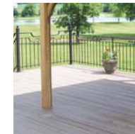
No floor (installed on existing floor)
